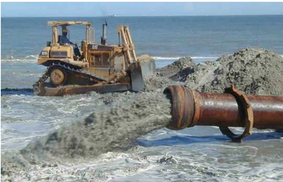
Figure 17. Typical beach nourishment operation—a dredge pumps sand onshore while bulldozers distribute the new sand (photo credit: USACE)
