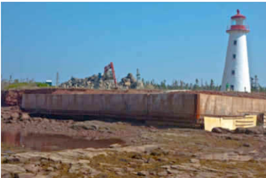
Figure 2. Seawall constructed to protect the Point Prim Lighthouse in Prince Edward Island. (photo credit: Don Jardine)
