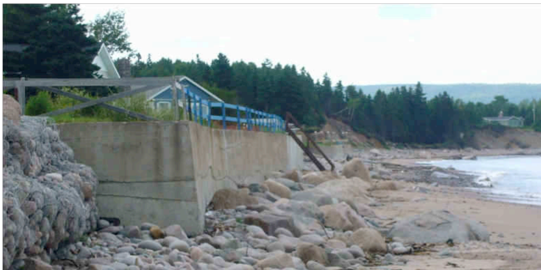
Figure 12. Three different types of residential shore protection are present along the west shore of Cape Breton: gabion baskets (foreground left), concrete retaining wall (centre) and armour-stone revetment (far distance).
