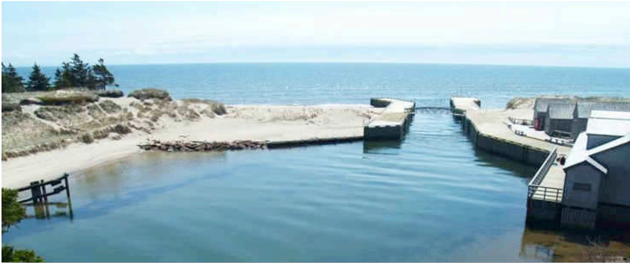
Figure 21. Hybrid protection at Basin Head, PEI: buried revetment covered with sand dune and marram grass.
