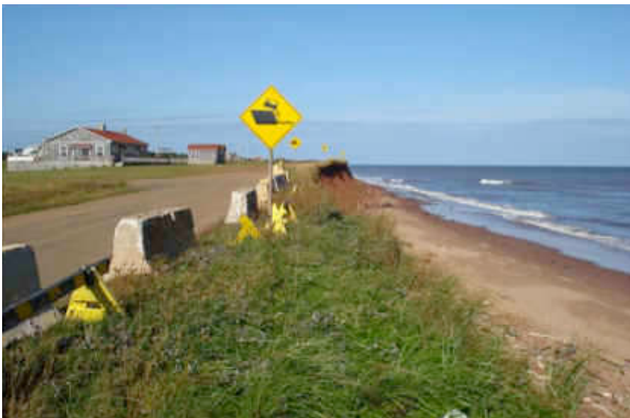
Figure 1. Shoreline retreat in North Lake, Prince Edward Island. Ongoing coastal erosion forced the abandonment of Cape Road. (photo credit: PEI Transportation and Infrastructure Renewal).
