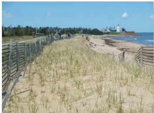
Figure 20. Panmure causeway May 2009, showing some armour-stone exposure and erosion of the rebuilt dune.
