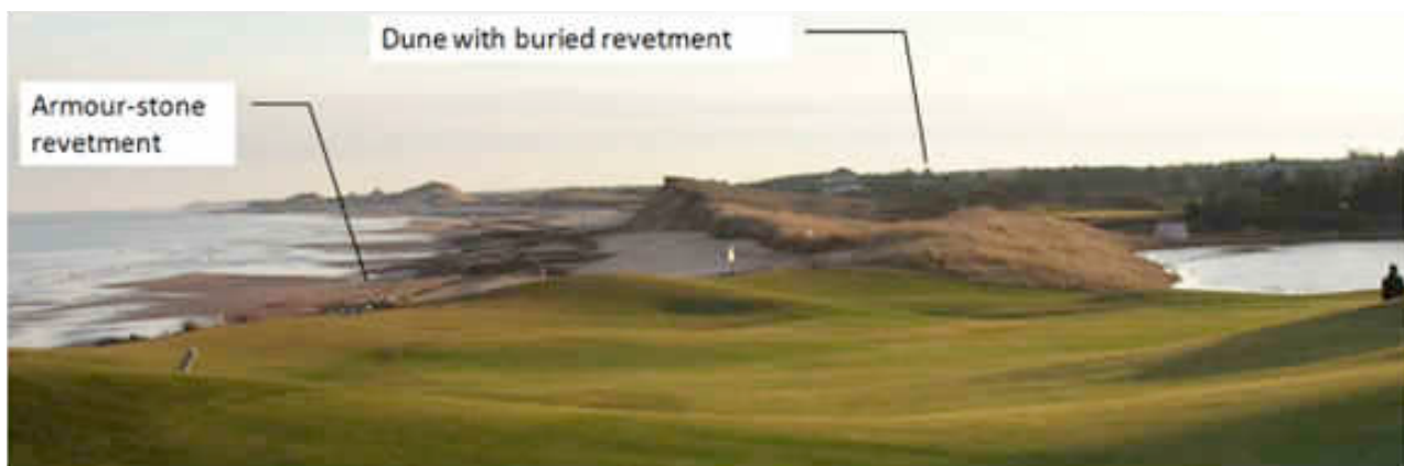
Figure 19. Fairway view with protection works hidden from view at Crowbush Golf Course four years after construction.
