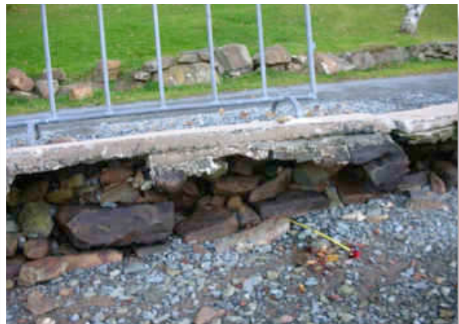
Figure 14. Seawall damage, Northwest Arm, Halifax.
