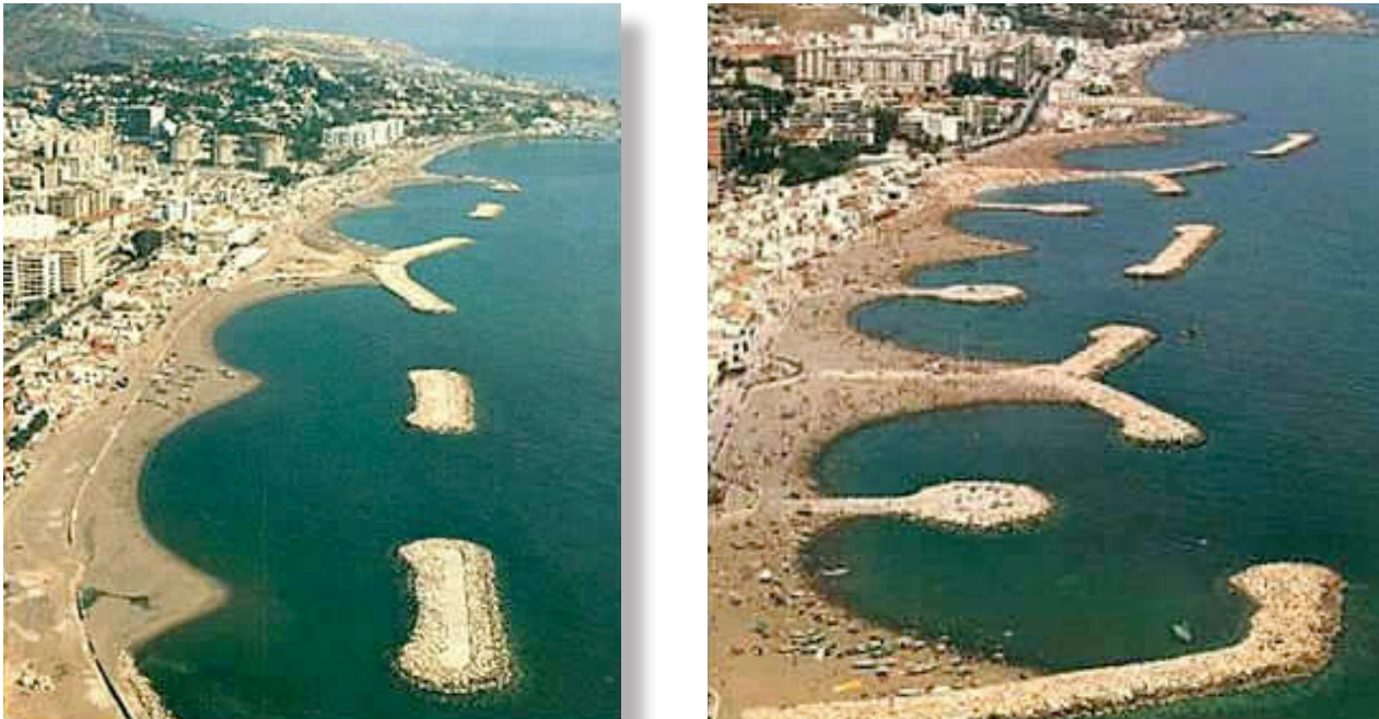
Figure 22. Examples of hybrid shore protection in Portugal using beach fill contained by artificial headlands and offshore detached breakwaters. (Dirección general de puertos y costas 1988)
